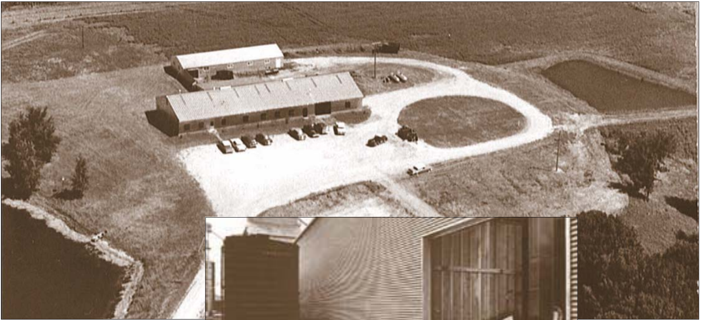
Original Humboldt plant
