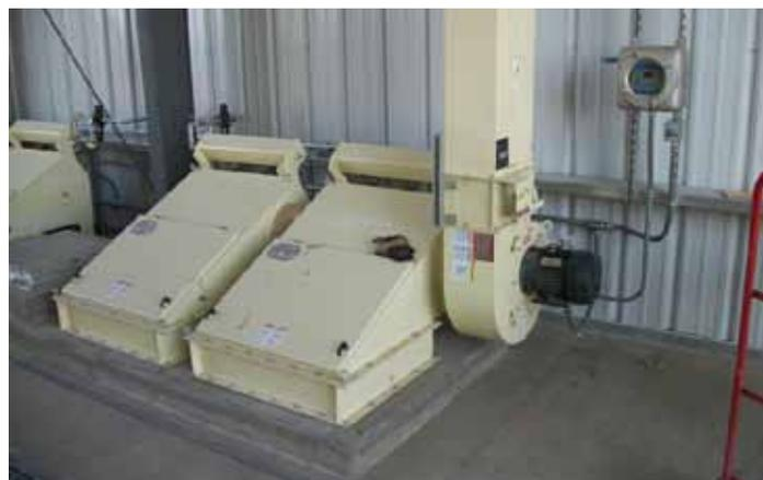
Point-of-use dust collectors allow for easy maintenance.
