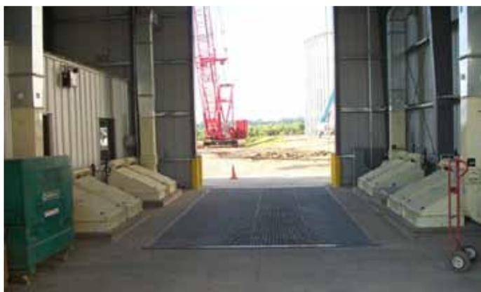
Point-of-use dust collectors capture nuisance dust while keeping product with the grain stream.
