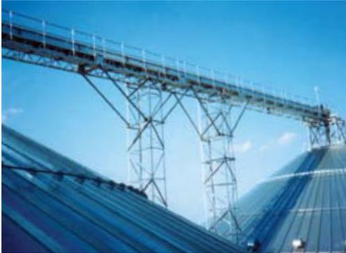
**Pre-Engineered Galvanized Steel Modular Conveyor Support Systems and Walkway**
