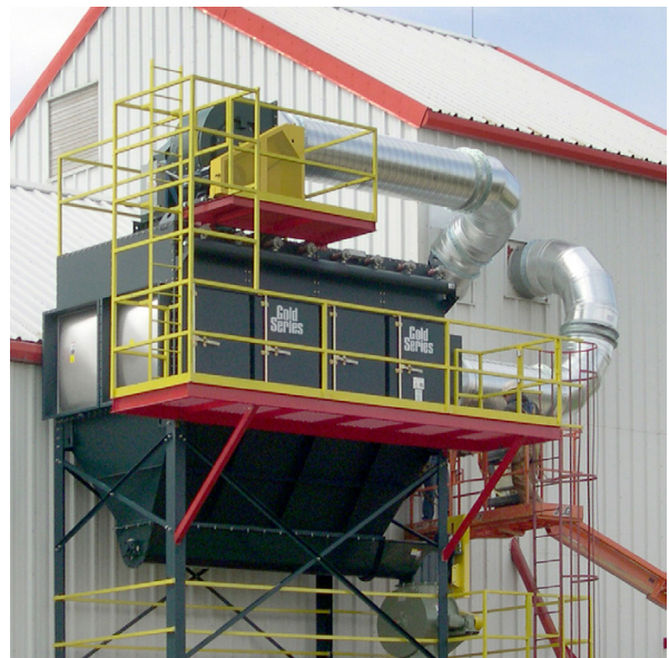
Dust collector at a corn shelling operation.
