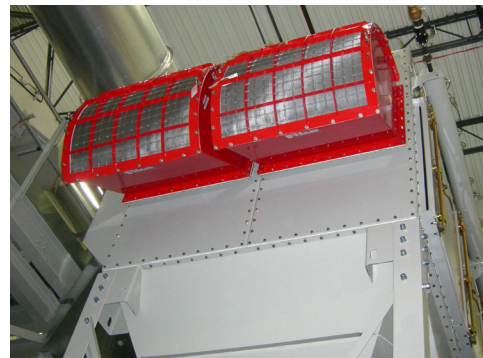
For dust collectors installed indoors, flameless venting provides a safe option to mitigate combustible dust explosions.
